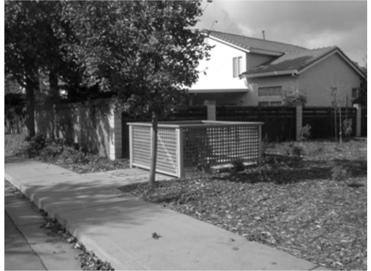
*Landscaping and Fencing adequately screen a device while maintaining required clearance and visibility.*
