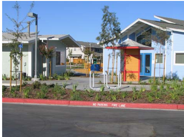
Moore Village Project
